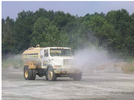
A water truck is used to keep dust at a minimum.
